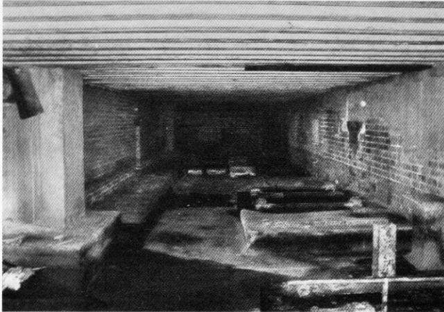
The void beneath Topshop in 2011.
